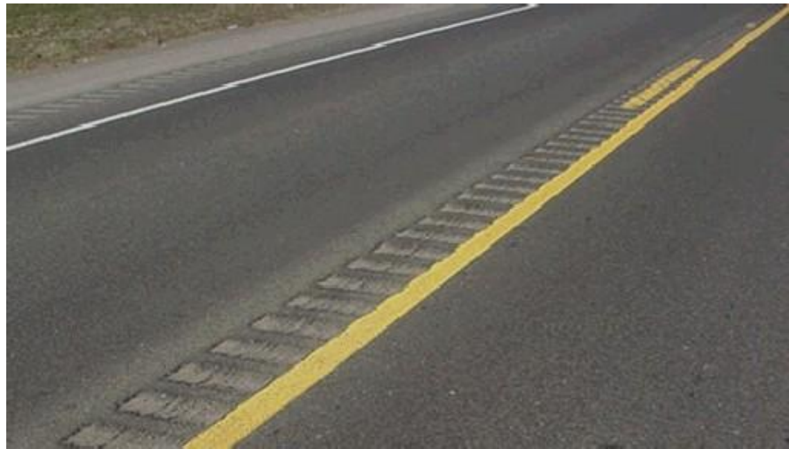
Center line rumble strip photo source: Transportation Research Board
